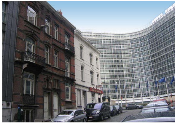
CCME office (red building on the left) in front of European Commission Headquarters (Berlaymont)
